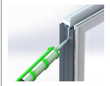
Apply a continuous bead of sealant to the other side of the structural mull groove that will set over the second windows nail fin.
