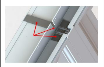
Seal both ends of the mull gaps with silicone the entire width of the frame covering any gaps and tool flat.
